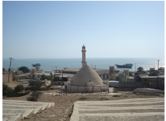
Figure 3: A water reservoir in Laft Historical Port, Qeshm Island
